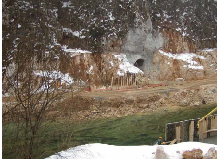
HE Lešće – ulaz u obilazni tunel
