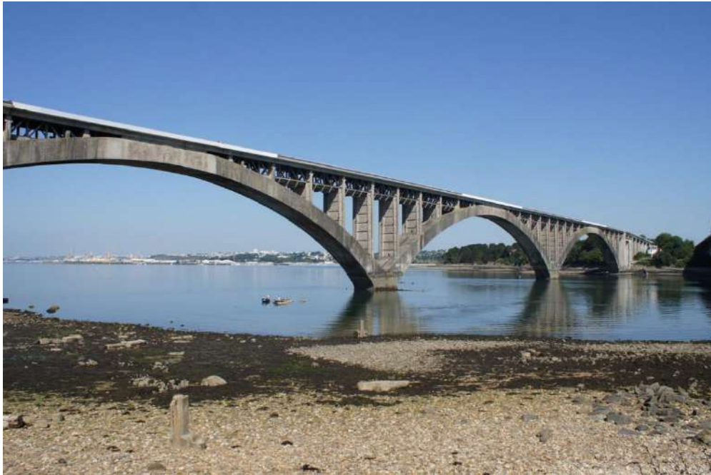
Slika 12. Most Albert Louppe ( https://structurae.net/en/structures/plougastel-bridge )
