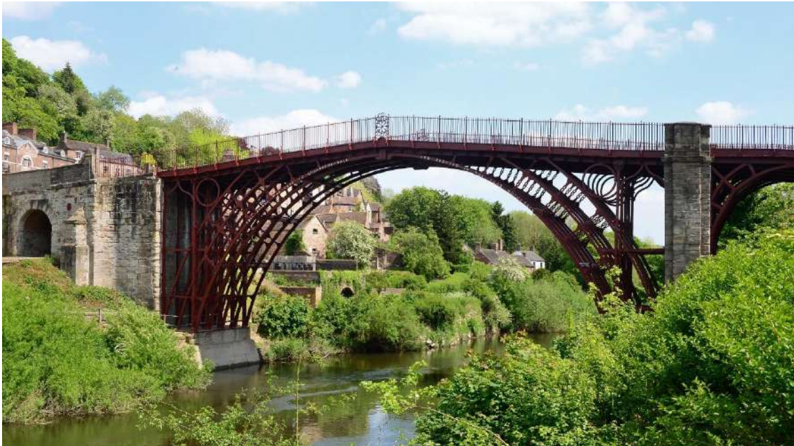
Slika 9. Željezni most preko rijeke Severn ( https://www.erih.net/i-want-to-go-there/site/iron-bridge-world-heritage-site )
