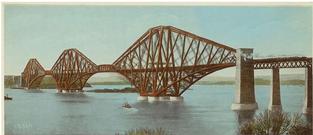
THE FORTH BRIDGE. THE LABOUR OF 5000 MEN (DAY AND NIGHT) FOR 7 YEARS. ENGINEERS—SIR JOHN FOWLER & SIR BENJAMIN BAKER. COST OVER CONTRACTOR—SIR WILLIAM ARROL. OPENED MARCH, 1890. £3,000,000 LENGTH, INCLUDING APPROACH VIADUCTS, OVER 1½ MILES. TWO SPANS OF 1710 FT. EACH AND TWO OF 690 FT. EACH. HIGHEST PART ABOVE SEA LEVEL AT HIGH TIDE, 361 FT. HEIGHT OF RAILS ABOVE SEA LEVEL AT HIGH TIDE, 157 FT. 8 INS. DEPTH BELOW WATER LEVEL, 91 FT. MATERIALS USED: STEEL: 54,160 TONS. CONCRETE: 64,300 CUBIC YARDS. GRANITE: 740,000 CUBIC FEET. CEMENT: OVER 21,000 TONS. ORDINARY STONE: 48,400 CUBIC YARDS. RIVETS: 6,500,000 = 4,200 TONS.
